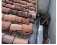
The following pictures correspond to the roof of the Foundation; in them you can appreciate the deterioration of the roof, product of the strong winter that affected us to all. Due to the winter and the lack of resources the roof has come being broken and leaks have been generated in the roof, which affect the structure that sustains it and in general the house.
