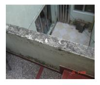
In these pictures you can appreciate the deterioration in which are the walls of the house, due to the strong winter that affects the region and to the deterioration in the roof, what allows that when raining the water it impacts with more force the walls and other areas of the house, the wood that sustains the roof and the wooden structures that it sustains both deteriorating.
