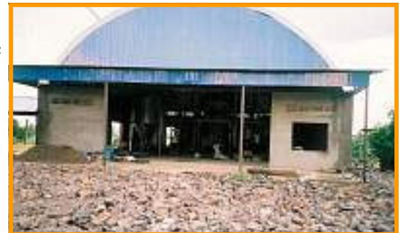
Rice mill — large rock had to be brought in to keep the 20 ton loads coming out of the mill from sinking.
