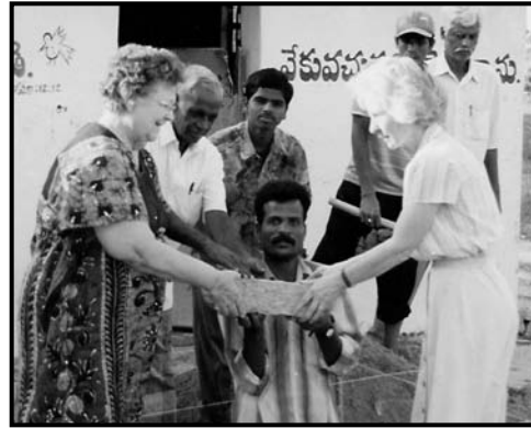
Geraldine (left) and Jan laying the first stone of the foundation for the new widow home.
