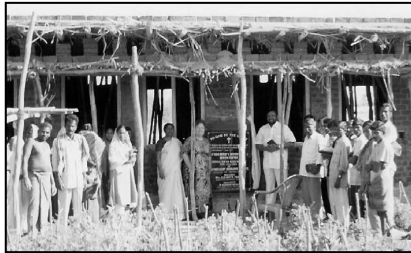
Widow home being constructed at Emmanuel Ashram, Chittoor, Andhra Pradesh, India.
